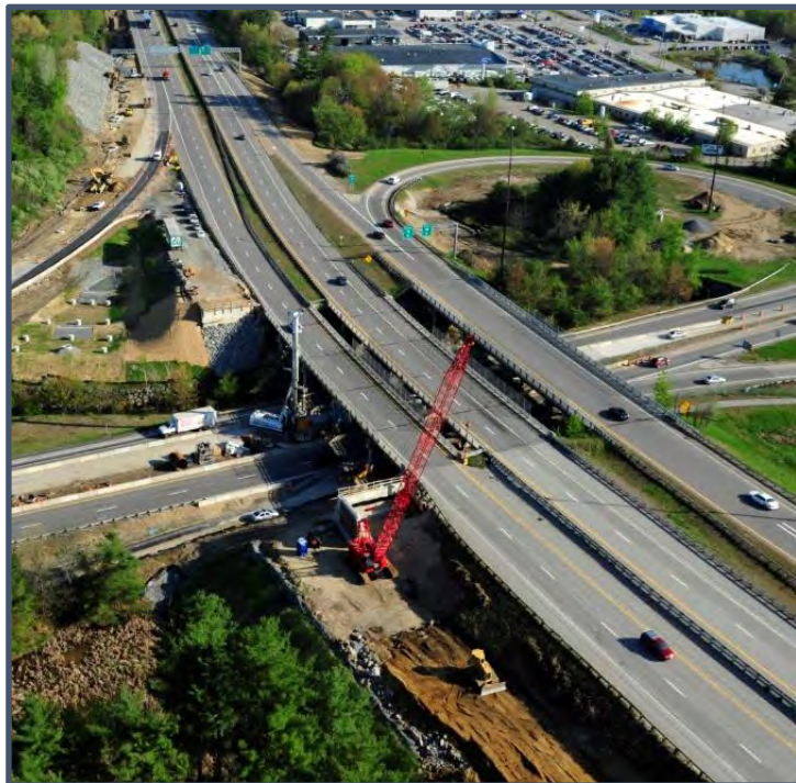
I-93 Bridges Under Construction in 2011
