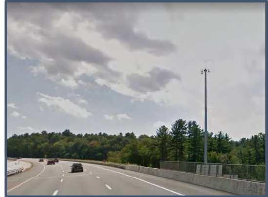
Existing ITS Camera at I-93/I-89
